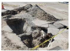
Now that the A/C has been fixed, there have been two water main breaks adjacent to the ITC loading docks. The County is taking bids to replace those two lines and re-concrete over them. Deliveries are now going to the warehouse in back and being unloaded with our forklift.
